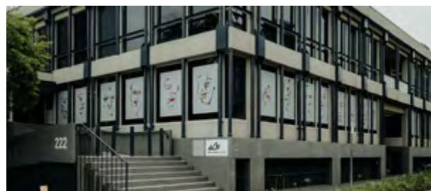
Front Up exhibition by Adam Knapper on AAV building, 2021. Photo by Raphael Recht.
